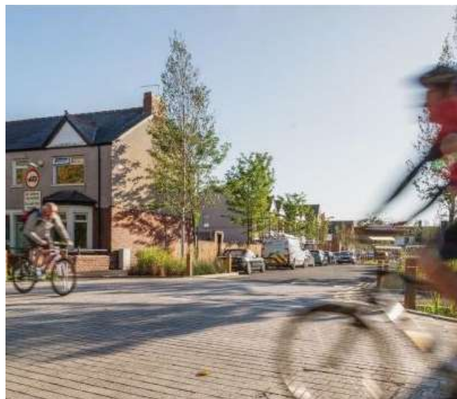
Inset 7.1: Rain gardens, tree pits and permeable paving integrated along a bicycle street, Grangetown Cardiff (source: Susdrain Case Studies)
