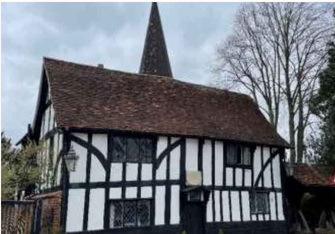
3 Traditional timber framed building, Churchgate Street
